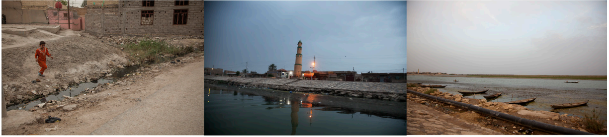
Exposed Sewage Pipes/ El Chibaish / Euphrates pipes
